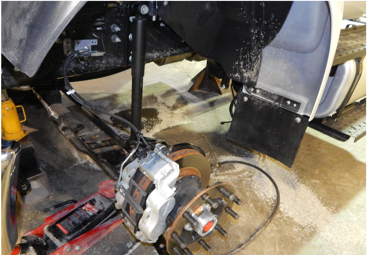
Drivers side ready for install
