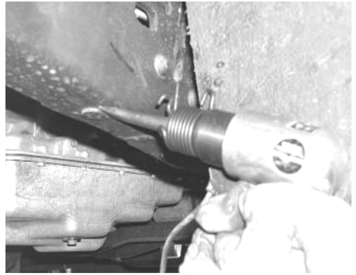
Removal of rivet with an air hammer
