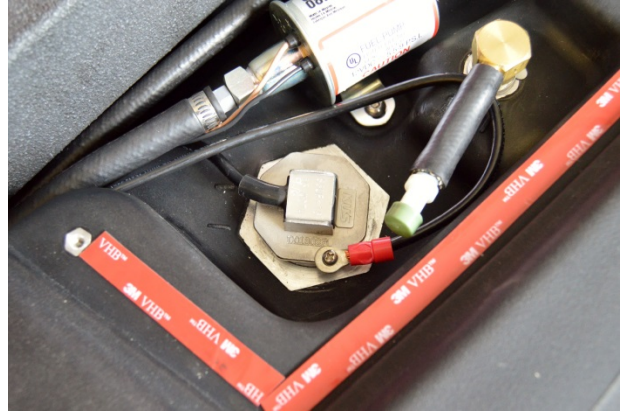
(Fig. 9) Showing grounding wire attached to the Electronic Level Sensor.
