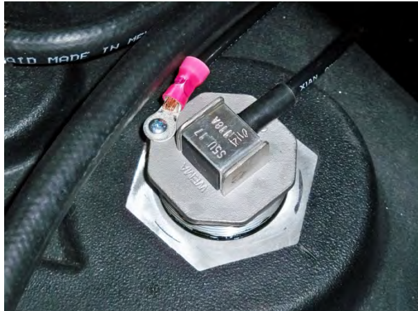
(Fig. 12) Attach ground wire to top of fuel gauge (shown above on the left), or the Electric Level Sensor shown above, right, depending on the model of tank being installed.
