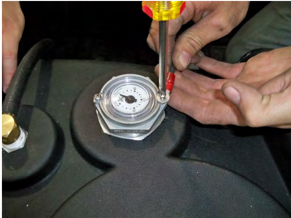
(Fig. 12) Attach ground wire to top of fuel gauge (shown above on the left), or the Electric Level Sensor shown above, right, depending on the model of tank being installed.
