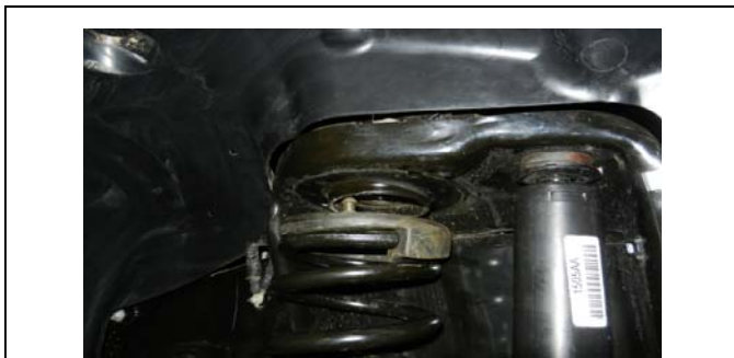
9. Lower the axle down to allow the front coil springs to be removed.
