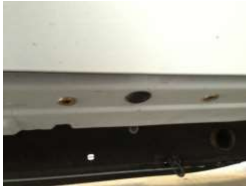
Nutserts properly installed
