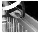
**Detail-A**: Apply the bulkhead seal by pealing off part of the seal's paper backing and sticking the pealed section to the bulkhead, slowly remove the paper backing as the seal is applied.
